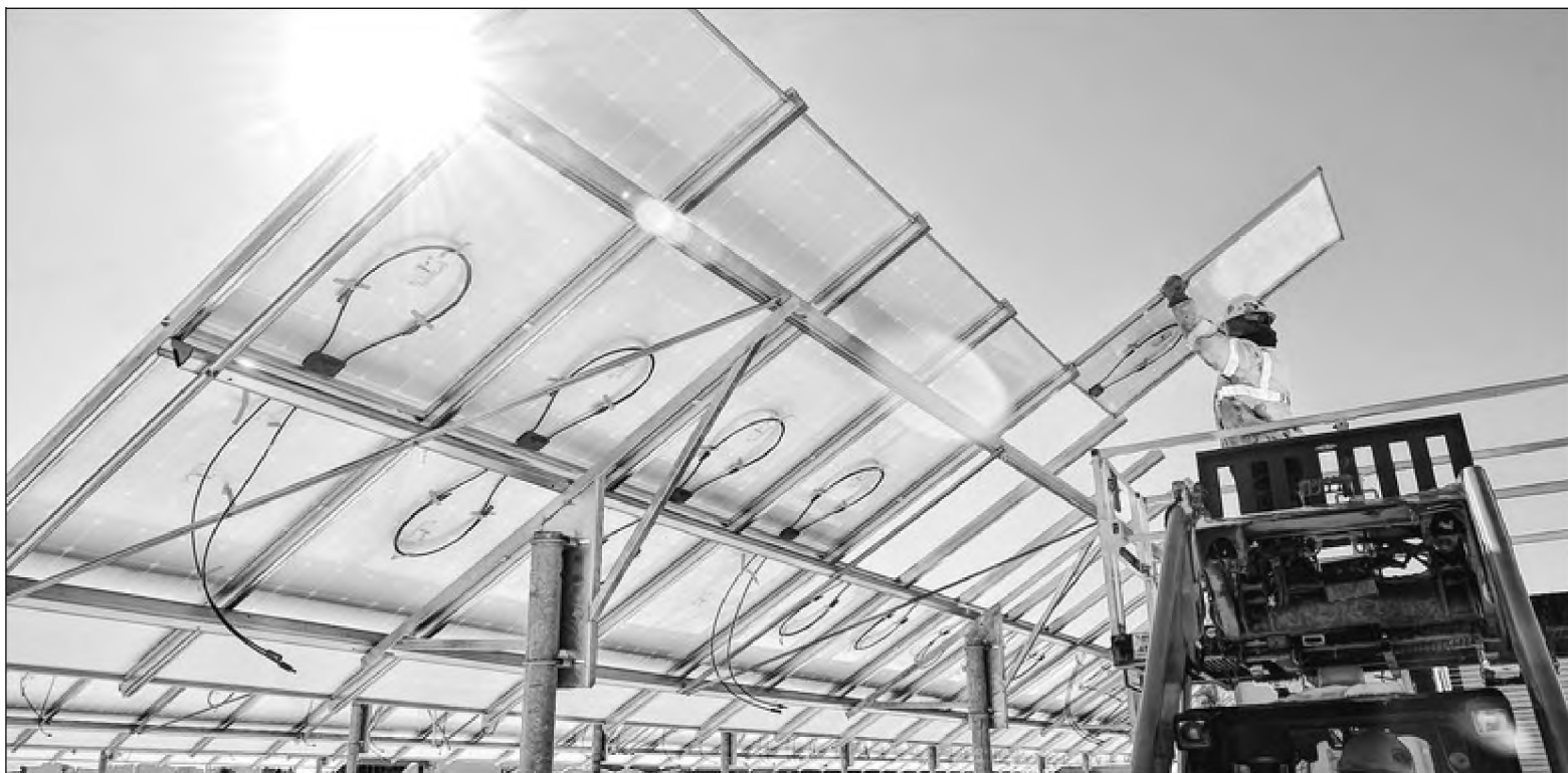
Chris Schear, an electrician for Ranck Electric, helps guide into place one of the 3,000 solar panels that are going up in Lyon Township along I-96 near Old Plank Road. Each panel should be able to generate, at peak-wattage, about 700 watts of electricity. PHOTOS BY JOHN HEIDER | STAFF PHOTOGRAPHER
