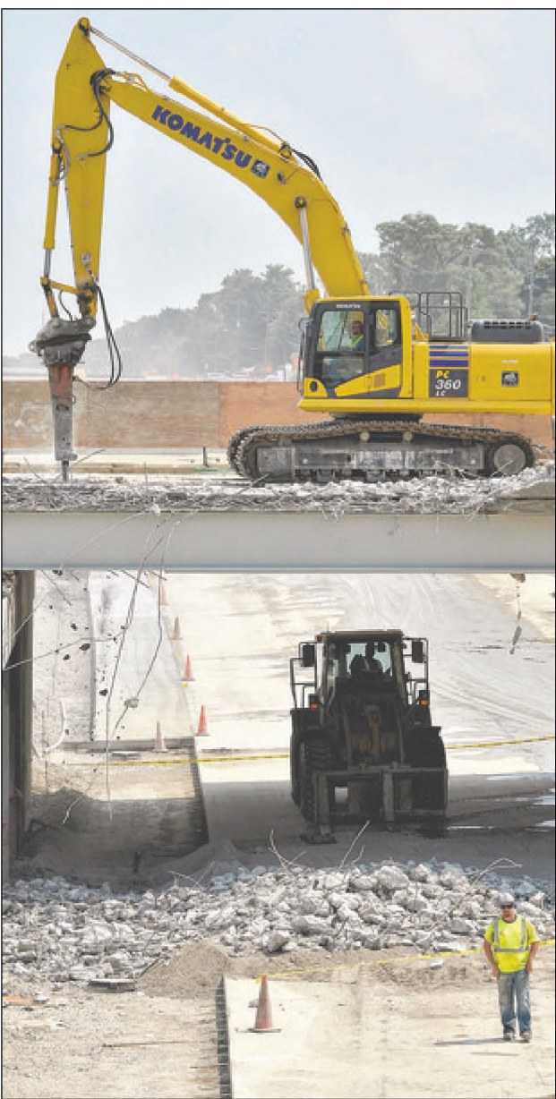
The road surface and side walls of the Beech Daly bridge are demolished, then rebuilt. BILL BRESLER | STAFF PHOTOGRAPHER
