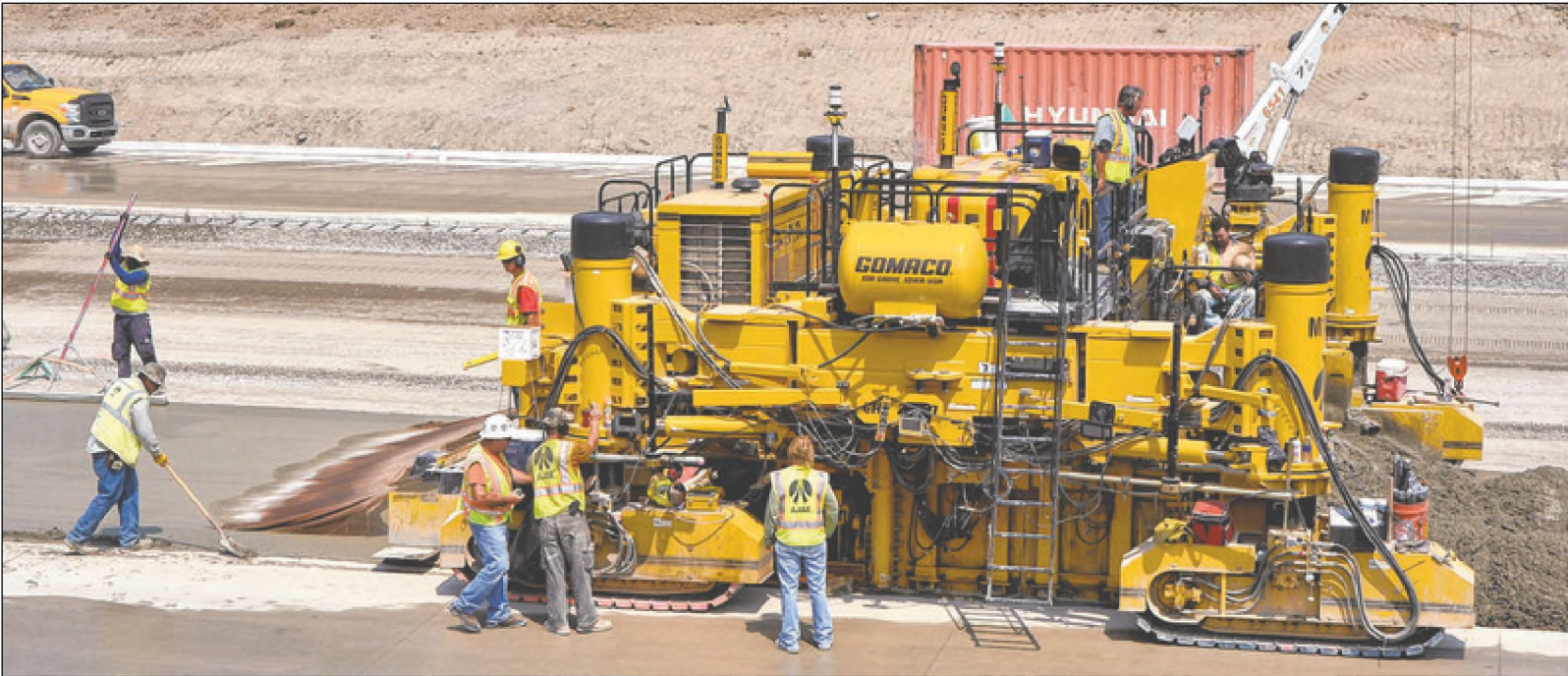
Miles of concrete are laid by machines like this. Mixed concrete is dumped in the path of the machine, which spreads and finishes the mix.
