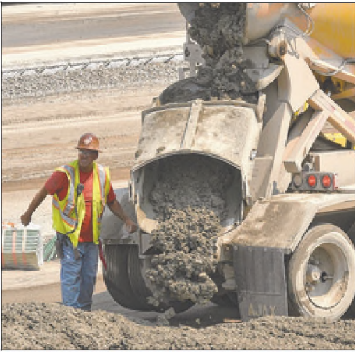
A constant stream of trucks dumps concrete that will become finished road surface, in a matter of minutes. PHOTOS BY BILL BRESLER | STAFF PHOTOGRAPHER
