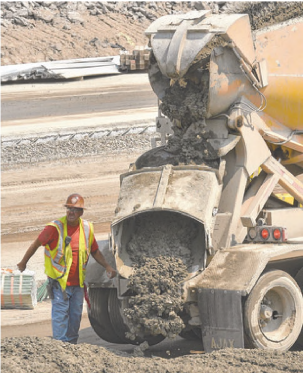
A constant stream of trucks dumps concrete that will become finished road surface, in a matter of minutes.
