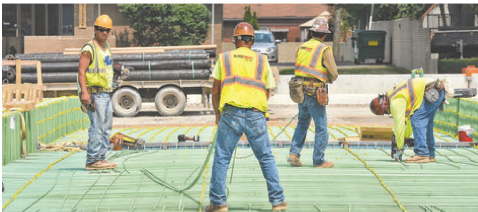
Reinforcing steel is laid before the concrete is poured for a new bridge surface.
