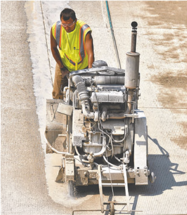
After the concrete sets, grooves are cut. When the road surface expands and contracts, the cracks should follow the grooves.
