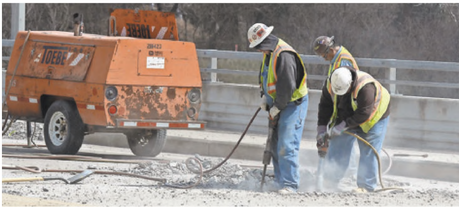
JOHN HEIDER | STAFF PHOTOGRAPHER The eastbound ramp over I-275 at Seven Mile is already closed as workers begin removing and replacing its road surface. The effort is part of the reconstruction efforts on the major highway that lies between Northville, Novi and Livonia and Farmington Hills.
