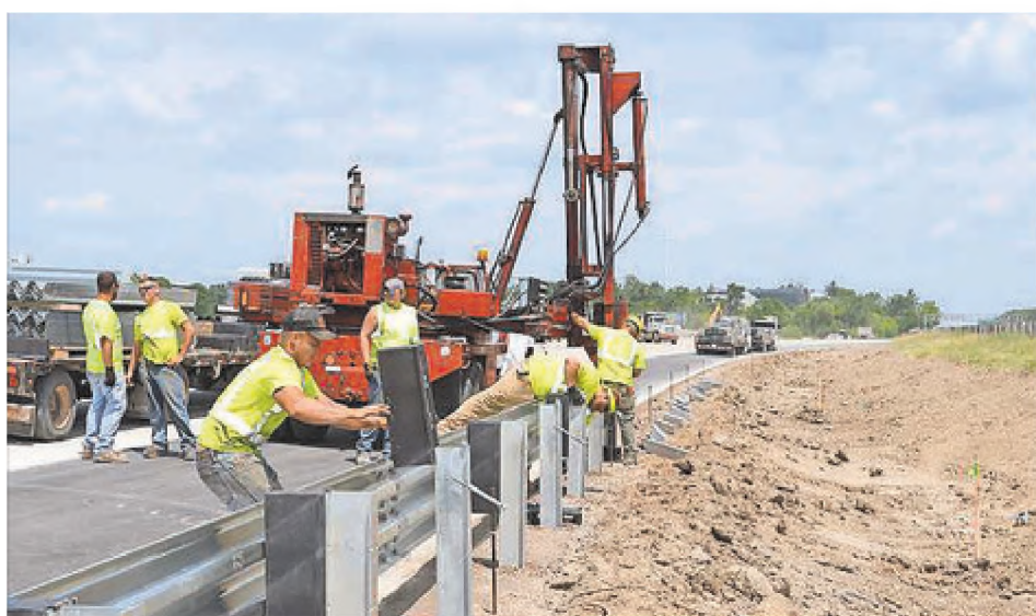
Crews work on the I-275 construction project earlier this summer.
