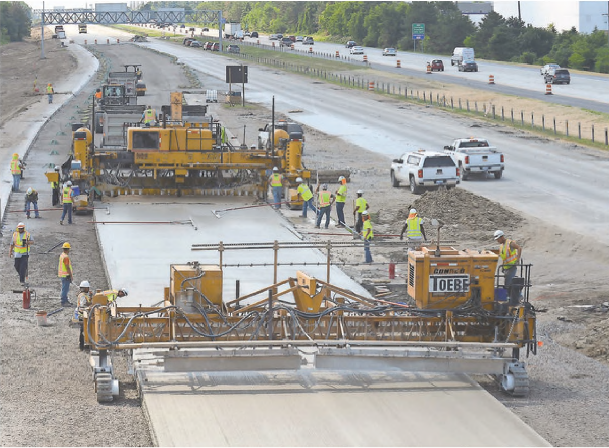
JOHN HEIDER | STAFF PHOTOGRAPHER Construction crews work on laying down fresh concrete pavement on I-275 northbound near the Ten Mile overpass on July 27. Work on the northbound lanes began in early July. The southbound lanes were finished first.
