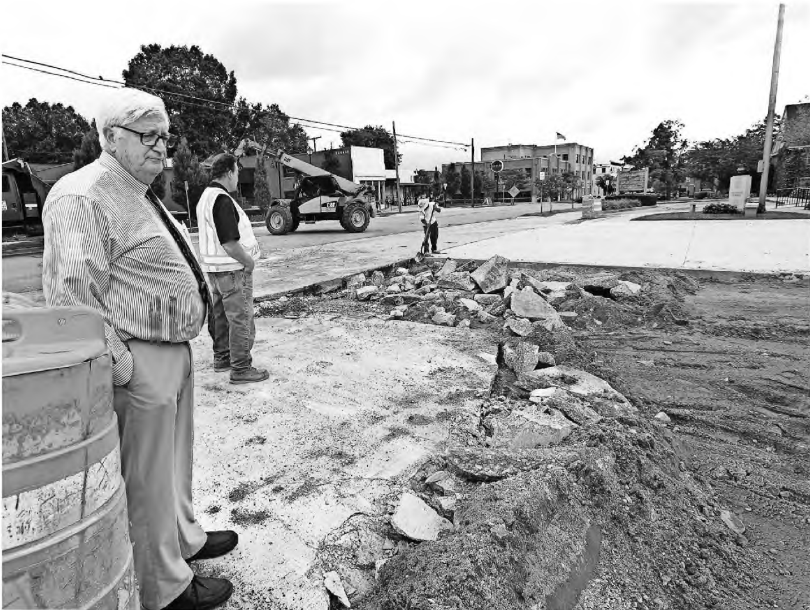
City of Northville Public Works Director James Gallogly takes a look at a project to replace the 8-inch thick concrete pad of the city's Main Street fire station July 24. One of the other station's outside concrete pads was replaced earlier in the year. It will take awhile for the new concrete to be able to bear the weight of the station's fire trucks.
