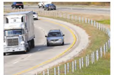
Cable barriers visible on I-96 near Portland are similar to what will be installed on a portion of I-96 near Williamston.
