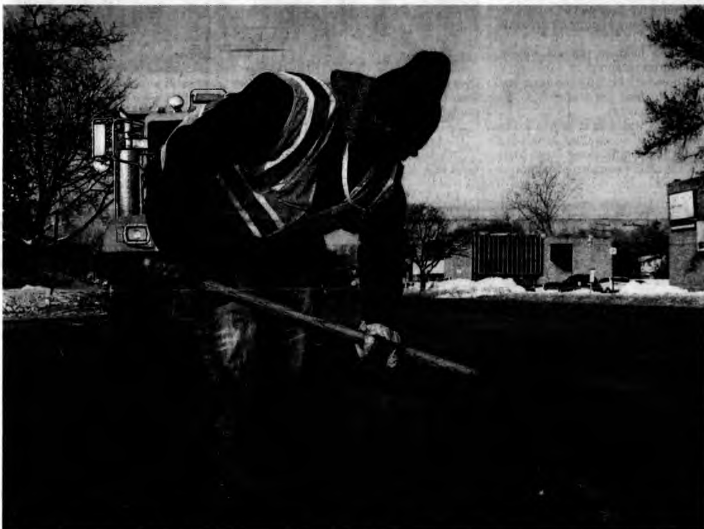
After filling the hole, Daimon Parker tamps down the patch with the back of the shovel blade. He knows the patch is temporary. Michigan's freeze-thaw cycle means that road crews never run out of work. BILL BRESLER | HOMETOWNLIFE.COM
