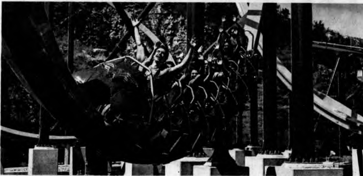
Nearly all roller coasters ride on two sets of rails. But Wonder Woman: Golden Lasso Coaster rests on a twisting, 15½-inch-wide steel monorail.
