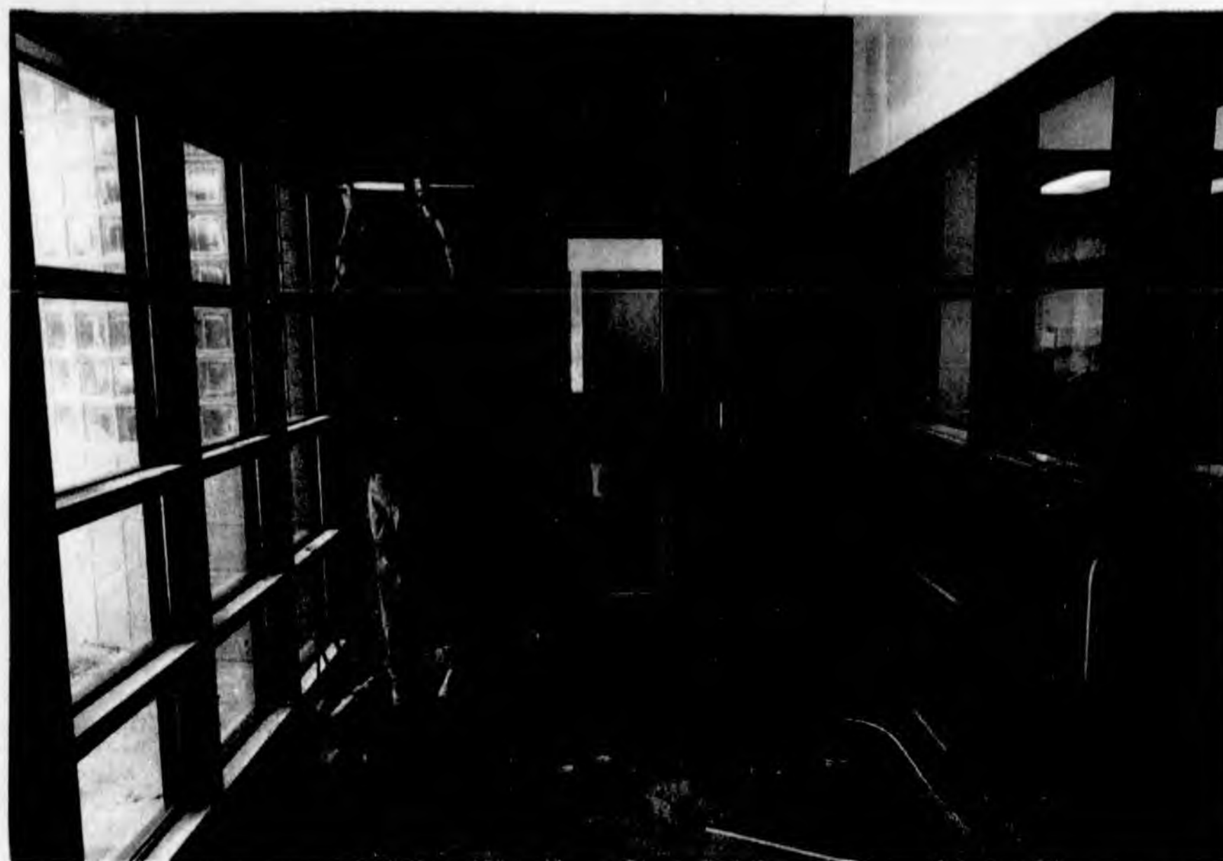
Jason Klinkovsky caulk the new double set of entrance doors installed at North Farmington High School. He works for Service Glass. BILL BRESLER | HOMETOWNLIFE.COM
