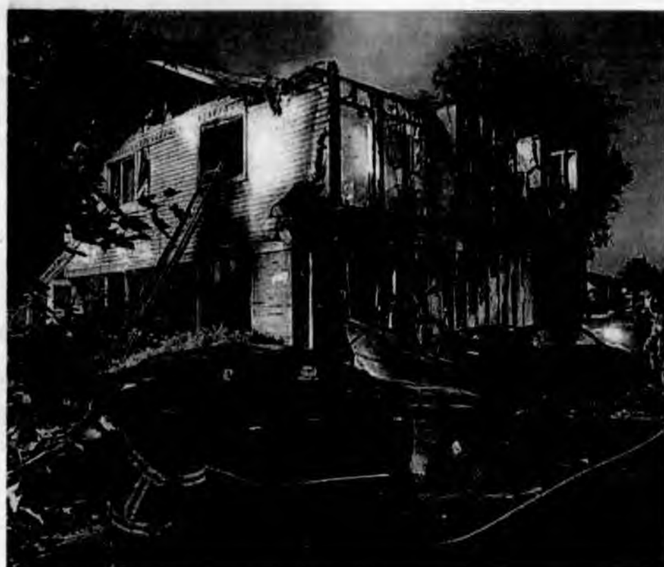
Fire, smoke and water damage wrecked the duplex and two vehicles. A home next door also sustained damage. PHOTOS COURTESY OF SOUTH LYON FIRE DEPARTMENT
