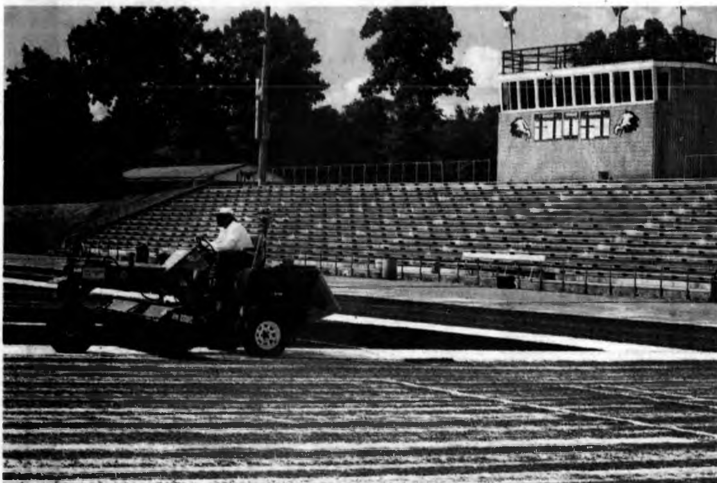
A renovation crew member spreads a cushioning layer of fine sand on Lakeland High's new artificial turf field July 14. PHOTOS BY JOHN HEIDER/HOMETOWNLIFE.COM
