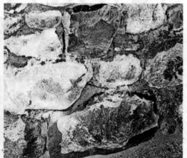
This 2017 photo shows how earth was seeping through the structure's original basement wall.
