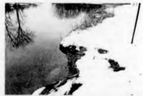
Milford will hope to stop erosion along the bank of the Huron River in its Central Park when it installs a kayak and canoe launch ramp.
