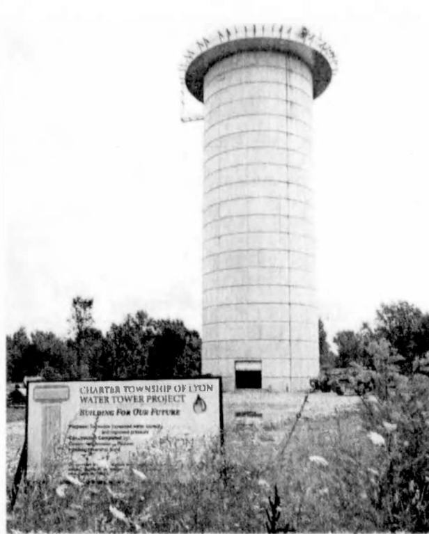
Construction continues on the Lyon Township water tower on Griswold near Nine Mile on July 22. A water tank will eventually be added to the top of the current structure. JOHN HEIDER | HOMETOWNLIFE.COM
