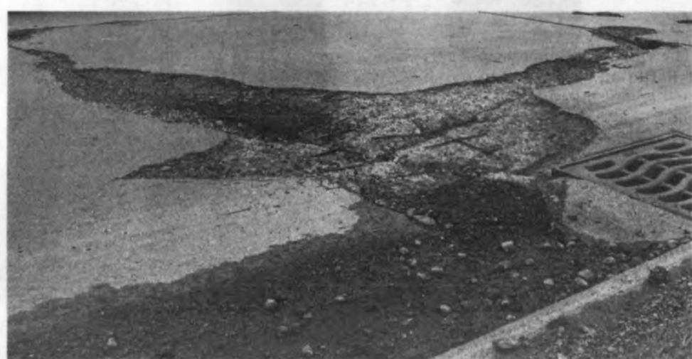
A collection of large potholes in the westbound lanes of Eight Mile Road between Haggerty and Meadowbrook. The exposed rebar can mean serious damage to tires. JOHN HEIDER/HOMETOWNLIFE.COM
