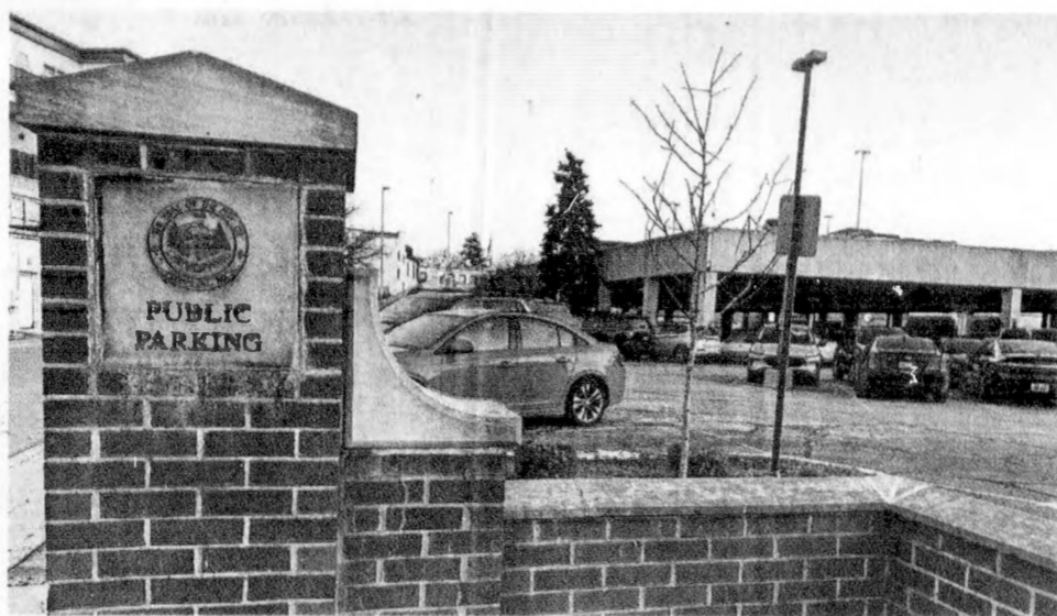
Many of Plymouth's parking lots, as well as the central parking deck, are in need of maintenance and repair. LAURA COLVIN/HOMETOWNLIFE.COM
