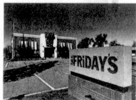
Developers plan to demolish the TGI Fridays at 44250 Ford Road to make way for a new Raising Cane's Chicken Fingers drive-thru restaurant.
